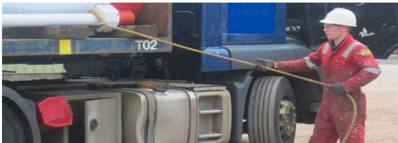
FIG 10.1. Tagline operator in correct working position. The rope is taut between the operator's gloved hands and the suspended load. The operator is at working distance, footing is stable, and the body position allows immediate movement in any direction.
