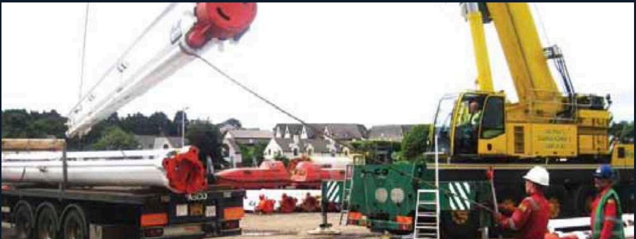
INDUSTRIAL CRANE OPERATION · LARGE LOAD SUSPENDED FROM MOBILE CRANE · TWO OPERATORS MAINTAINING WORKING DISTANCE
