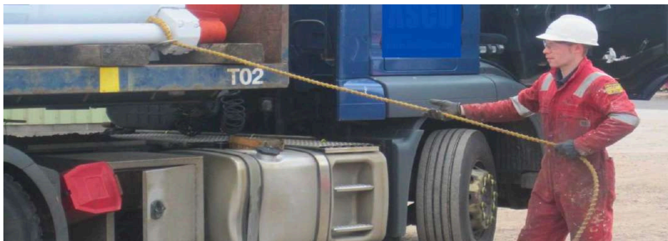
FIG 7.1. The yellow tagline is traceable from the operator's hands to the load attachment point. This visibility allows all members of the lift team to read the tagline's path and the operator's separation from the suspended load at all times.
