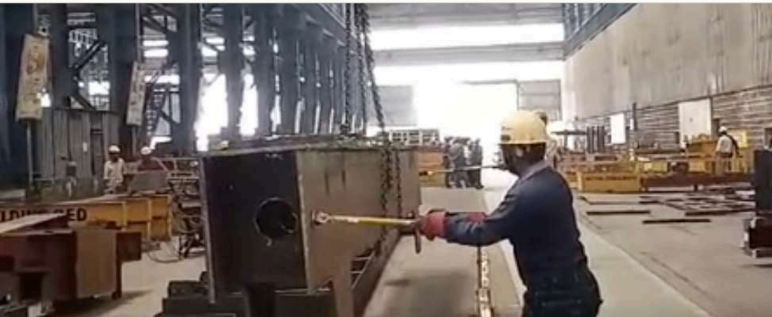
PSC Load-It® magnetic tool — guiding a suspended fabricated steel assembly, final positioning phase
